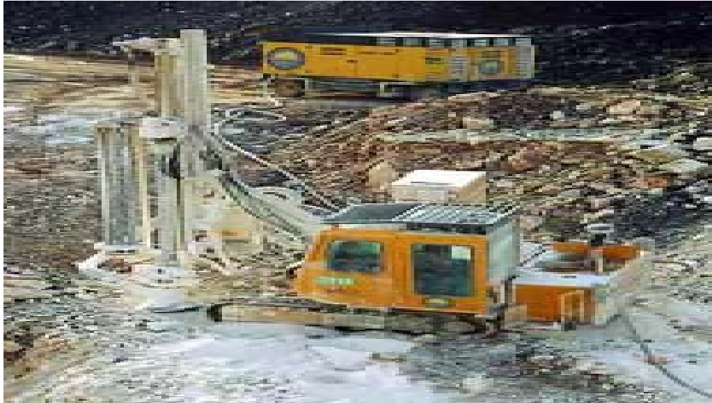
Plate 2: A machine drilling holes for blasting
