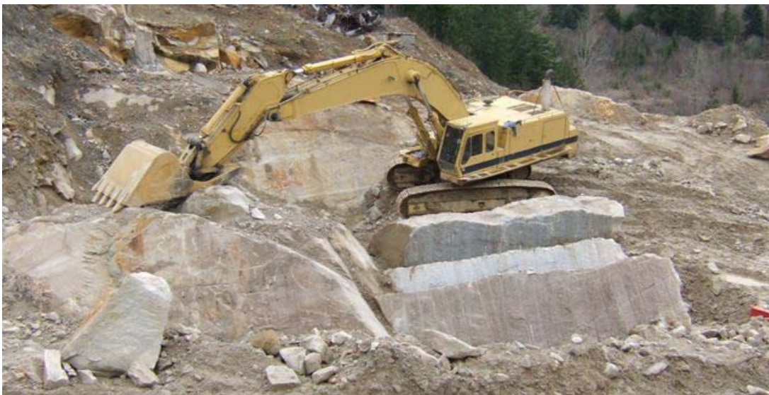
Plate 4: Caterpillar E650 moving quarry blocks downhill
