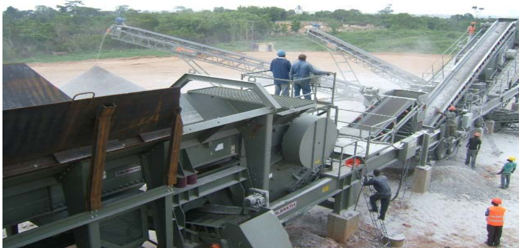
Plate 7: Conveyance of rock particles on conveyor belts at GHACEM Quarry
