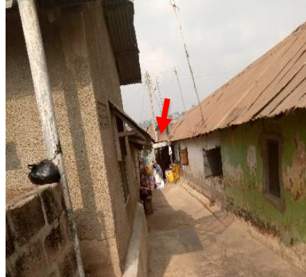
b. An outlet located in the alley
