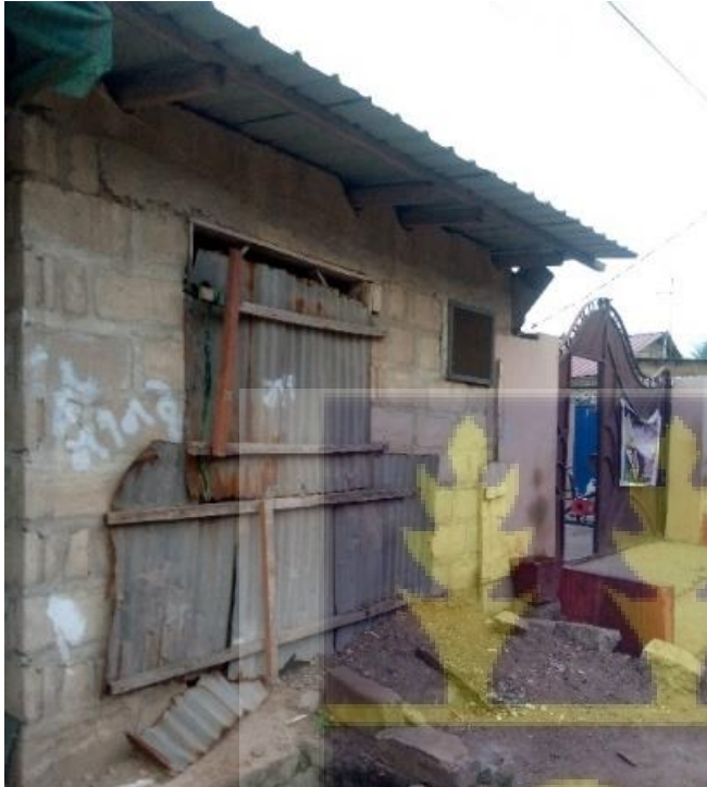
Figure 4.6: Uncompleted building extension for a retail outlet in Abelemkpe
