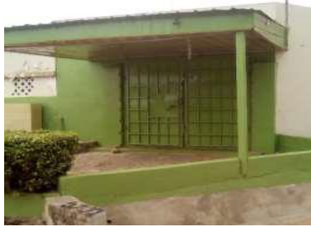
a. Concrete building outlet
