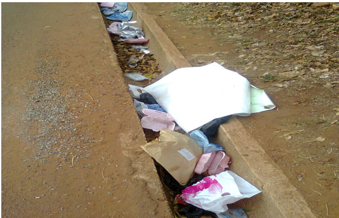
Plate 4.1 Rubbish blown into the gutter by wind
