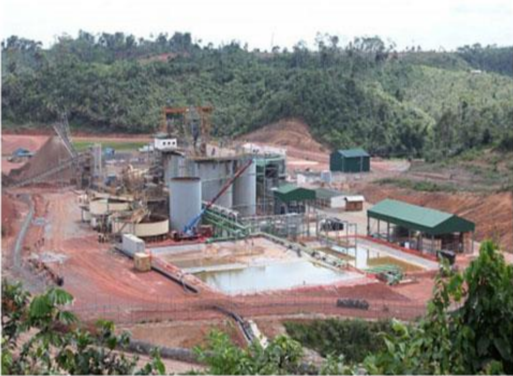
PLATE 1: Plant site in the study area
