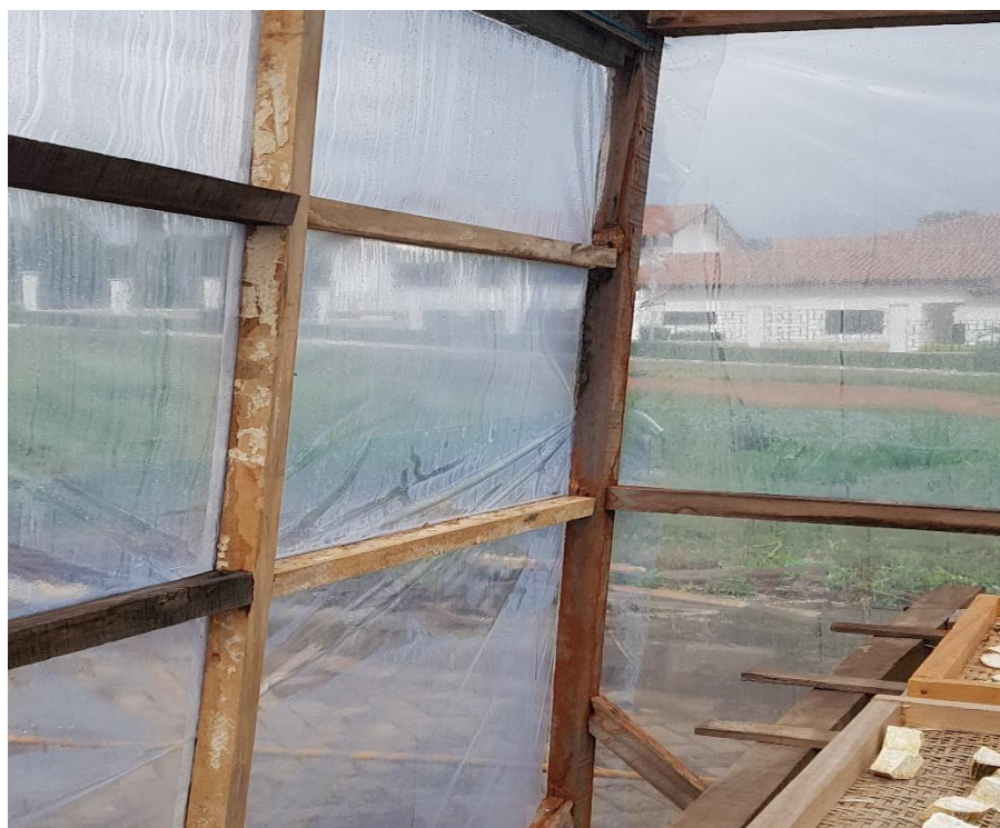
Illustration 20: Accumulation of moisture on the surface of the polycarbonate sheet inside the GSD
