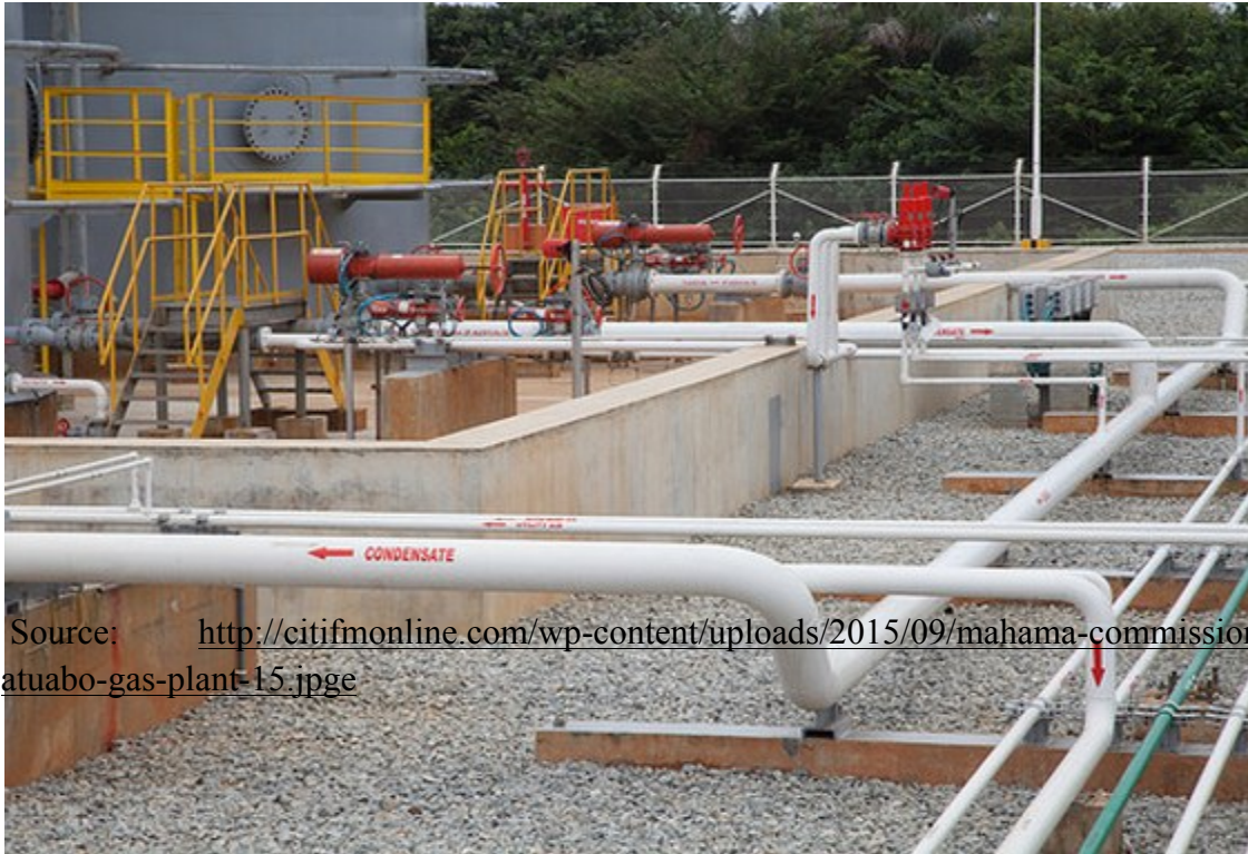
Figure 2: Atuabo Gas Processing Plant
