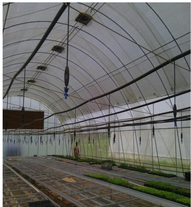
Plate 9: Sprinkler system
