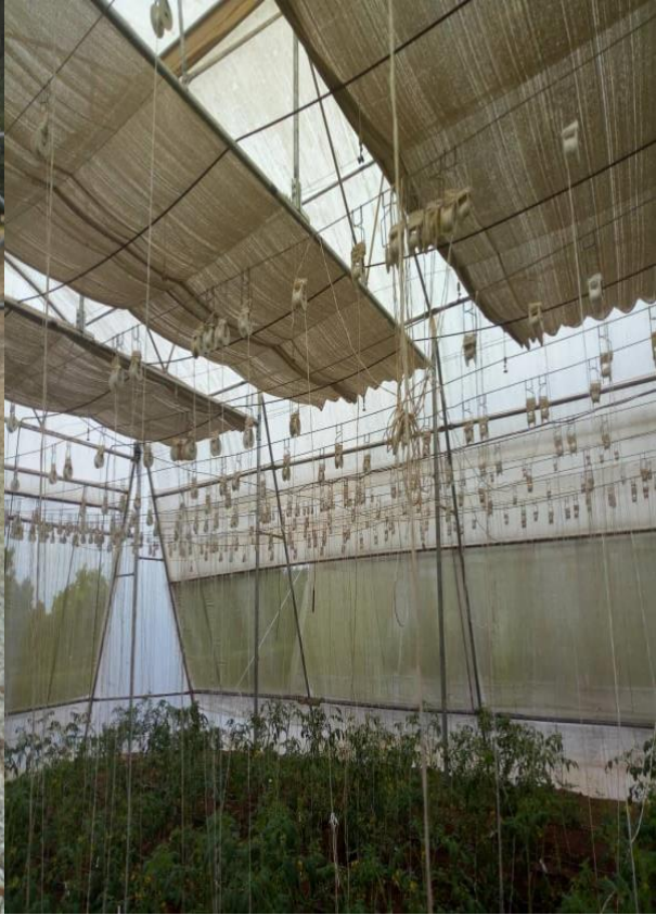
Plate 33: Sprinkler system and plant
