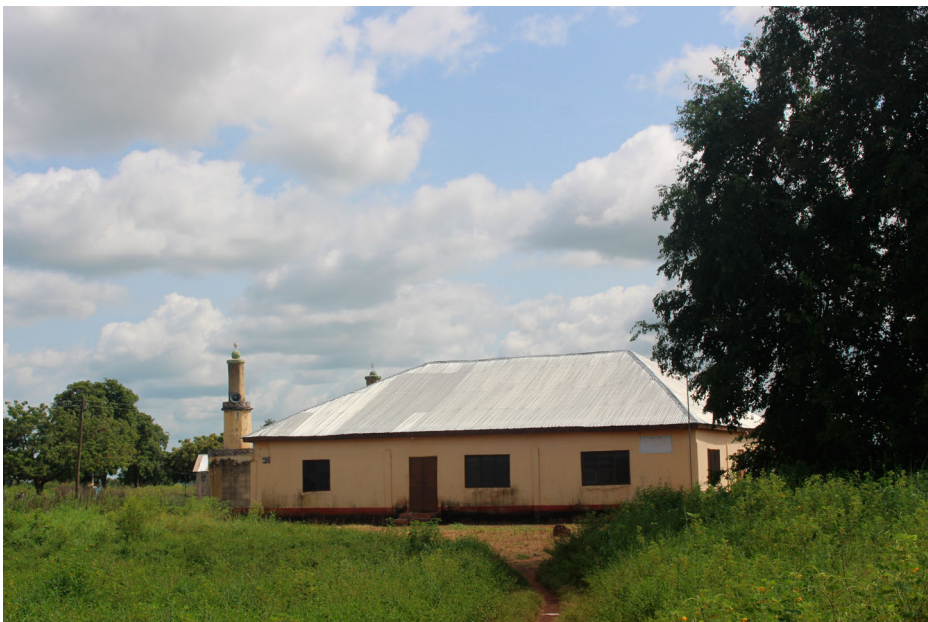
Figure 7. The Mosque in Gbabshe reflecting the transitioning from traditional earth buildings to cement-based and metal roofed building as a sign of modernity. Photograph taken by the author, 2019.
