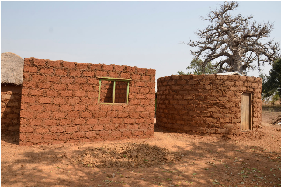
Figure 4. New buildings under construction. Photograph taken by the author, 2019.
