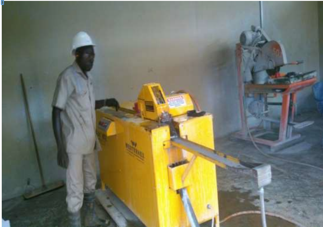
Figure 4: Mechanized core cutting process by DrillCorp
