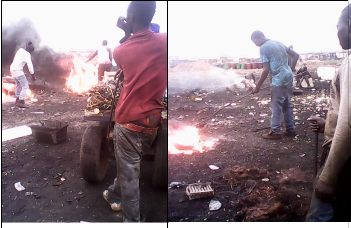
Plate 4.1: Burning of Sheathed Wire at Agbogbloshie to Harvest Copper
