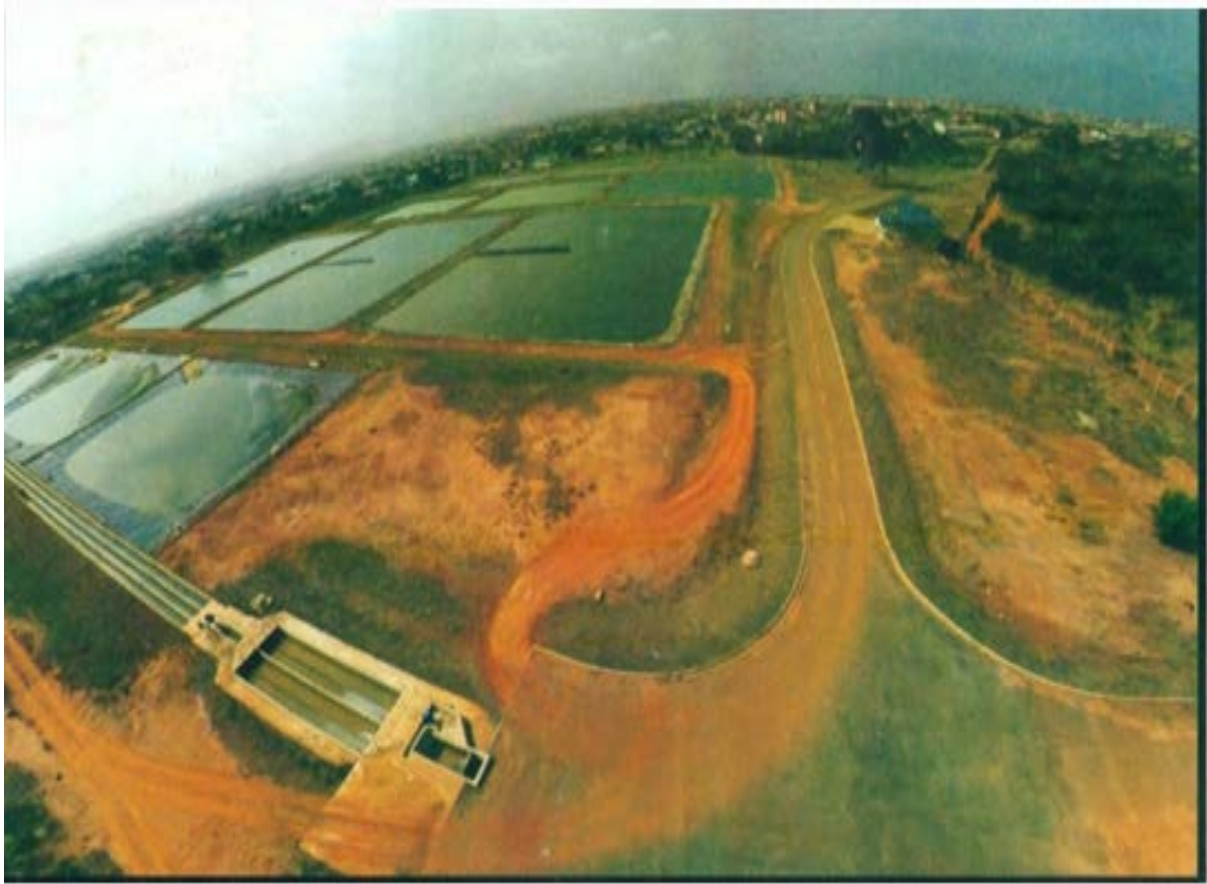
Figure 2: AERIAL VIEW OF THE SAMPLING SITE
