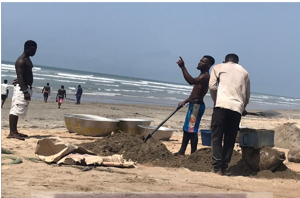
Plate 3.4: Indigenes of Half-Asini mixing beach sand and adhesive for construction purposes.
