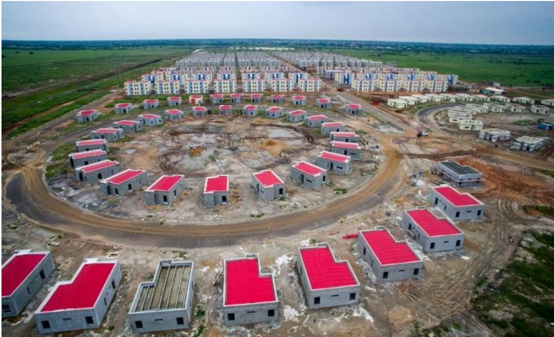
Plate 5: Abandoned Saglemi housing project Source: Fieldwork, 2020.
