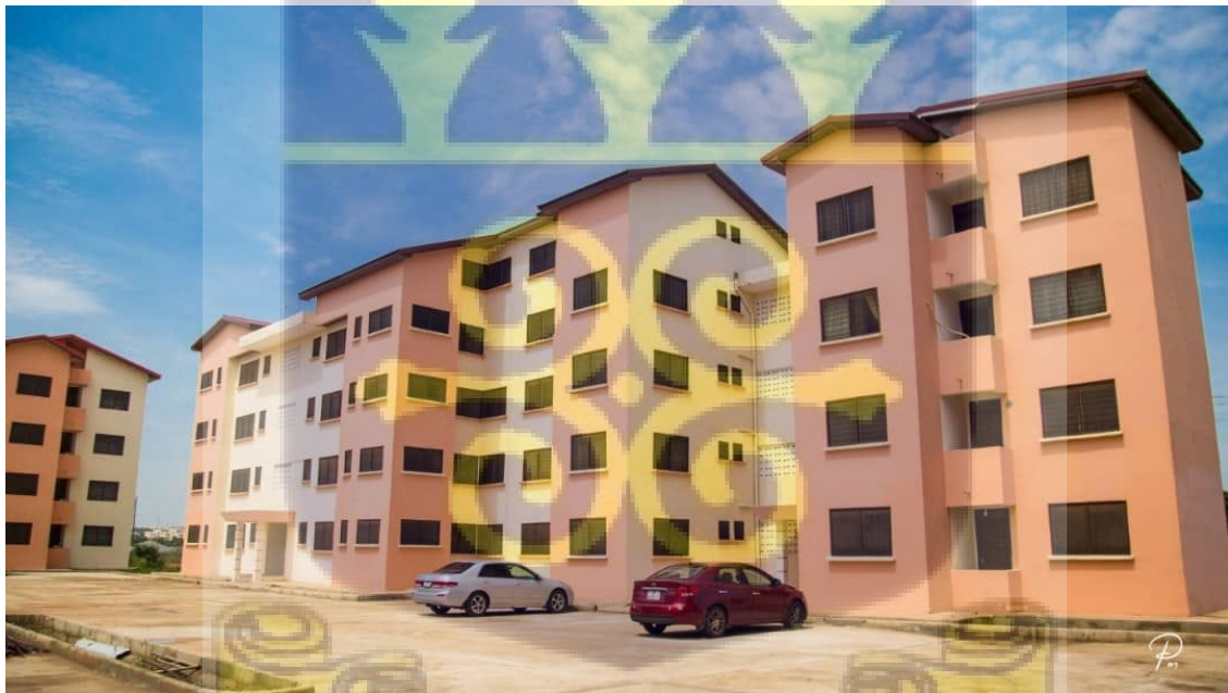
Plate 4: Completed portion of the Kpone affordable housing Source: Fieldwork, 2020.
