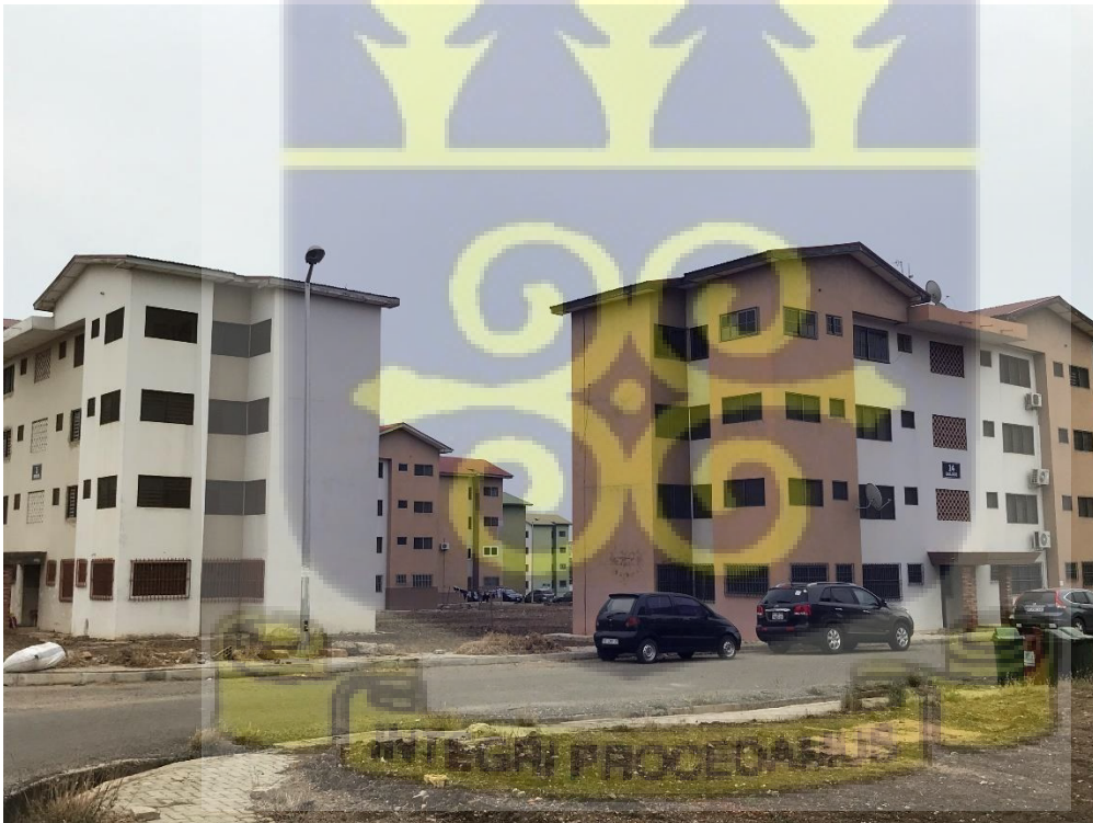
Plate 2: Portions of newly completed Borteyman affordable housing Source: Fieldwork, 2020.
