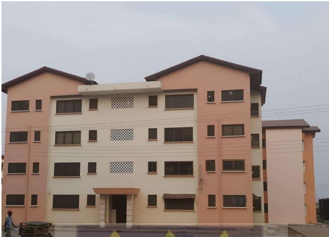
Plate 3: Completed portion of the Kpone affordable housing Source: Fieldwork, 2020.
