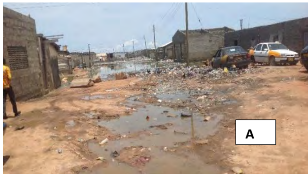
Before street and drain construction, Glefe Image A was taken in April 2015
