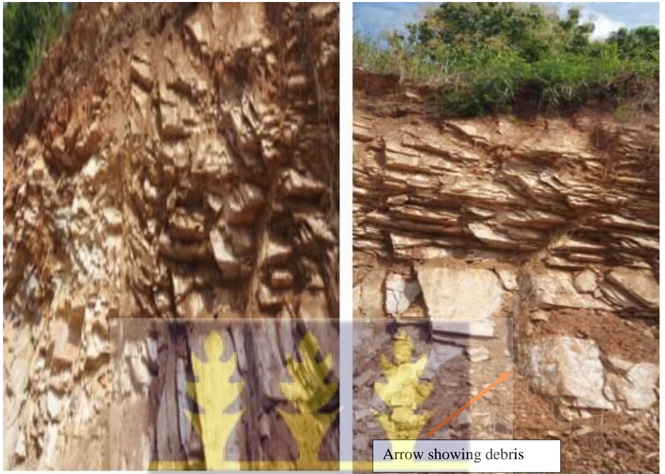
Plate 2: Debris slide as a result of slope excavation in Aburi
