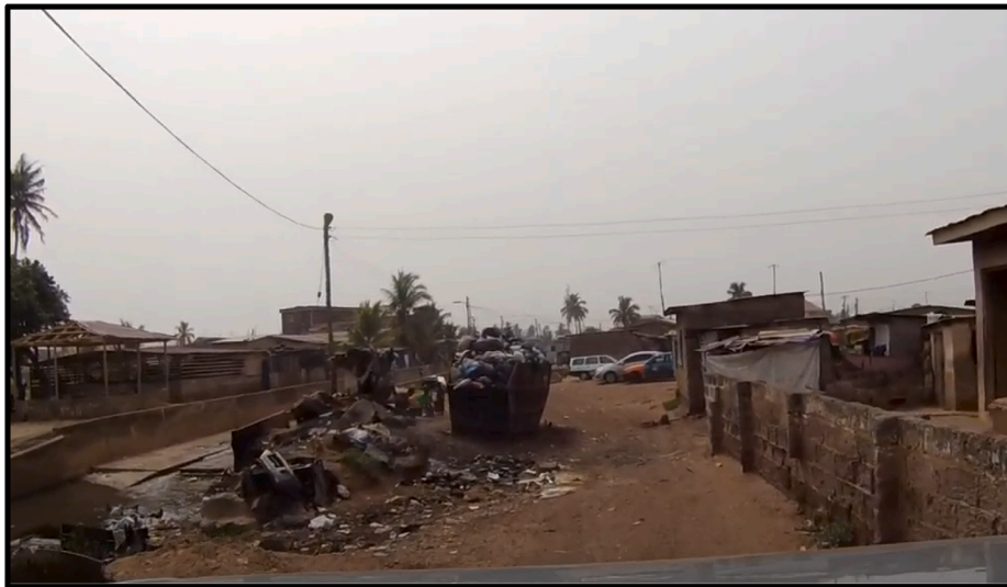
Fig. 10. An example of an overflowing dumpster located close to residential units and an open drain.
