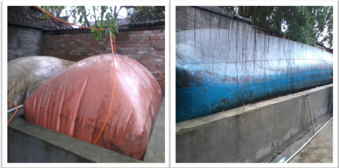
Figure 2-9: Soft polymer digester Source: (BIOMA P. R. C., 2013)
