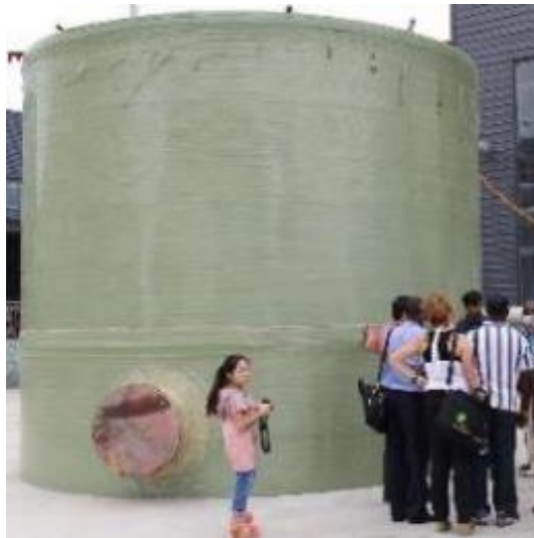
Figure 2-10: High rate digester Source: (BIOMA, P.R. C., 2013)
