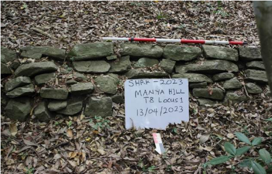
Figure 27: A preserved building foundation (photo by Odarkor Ankraah-Addison, 13/04/2023).
