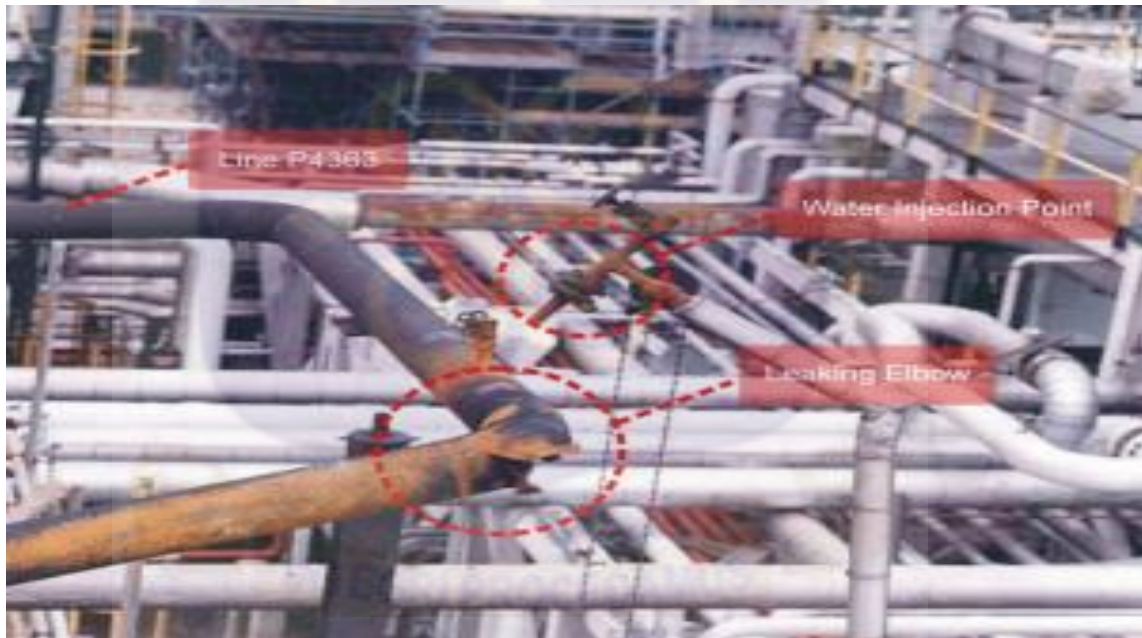
Figure 1.4: Mixing Joints in Piping Network
