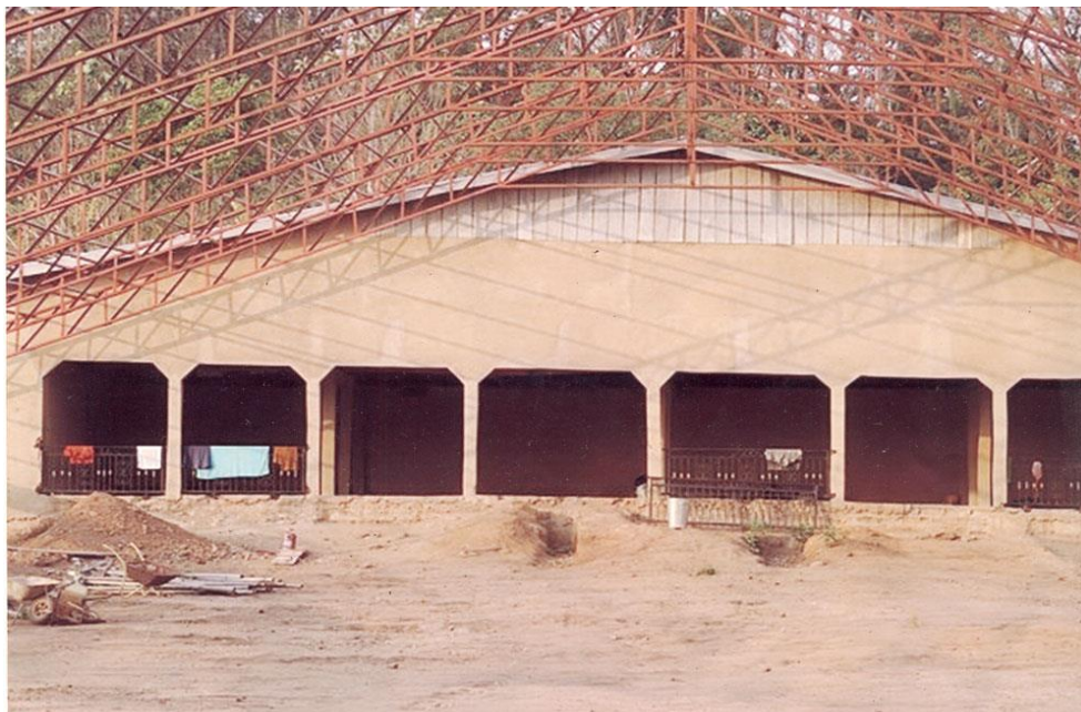
Picture 5: Dormitories attached to the auditorium
