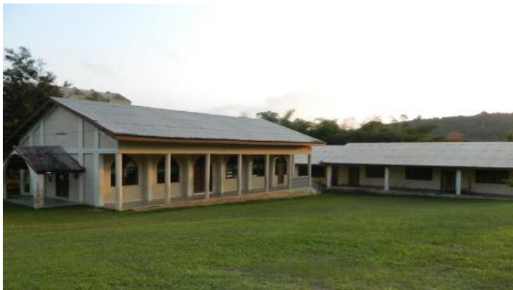
Picture 13: The chapel at Azani with a hostel behind it.
