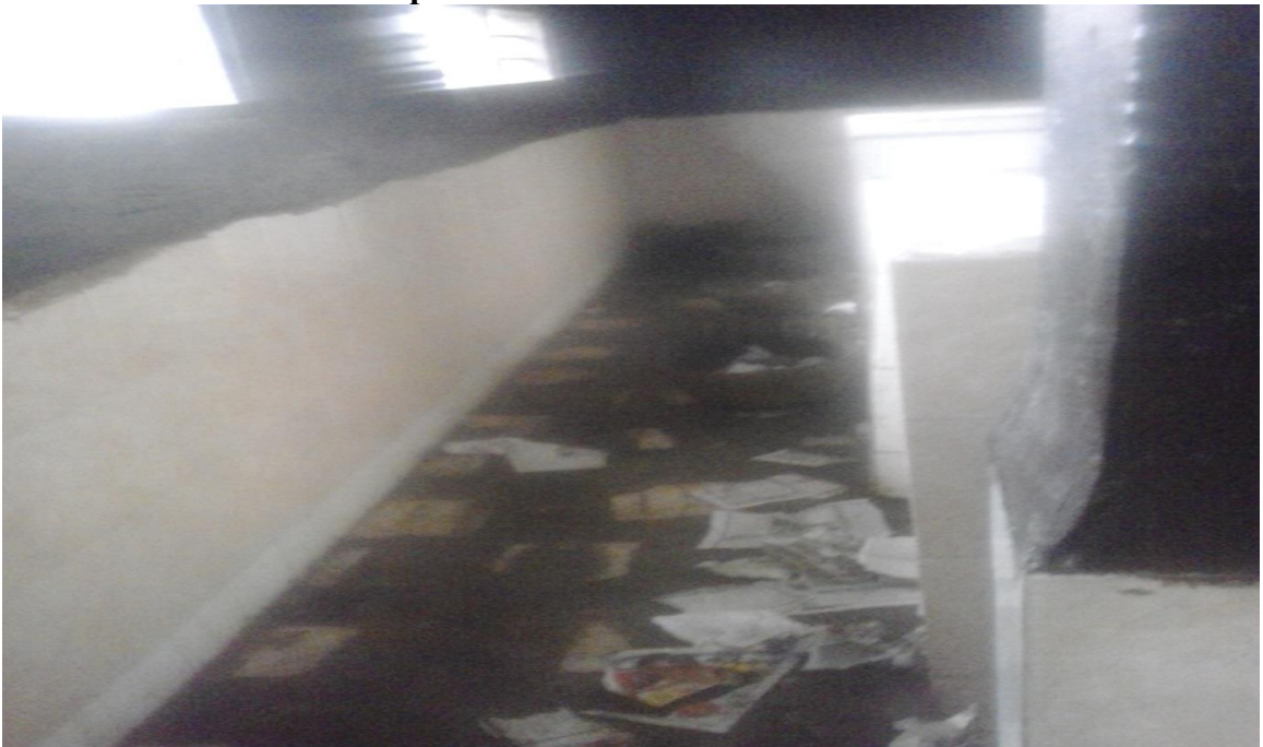
Picture 7: Corridors of the public toilet
