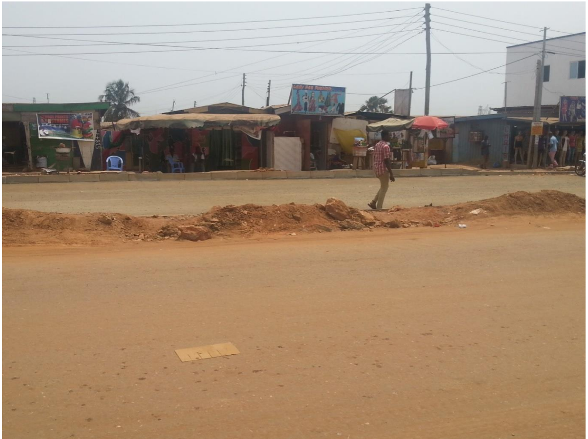
Picture 5: Abandoned road construction in Ashaiman
