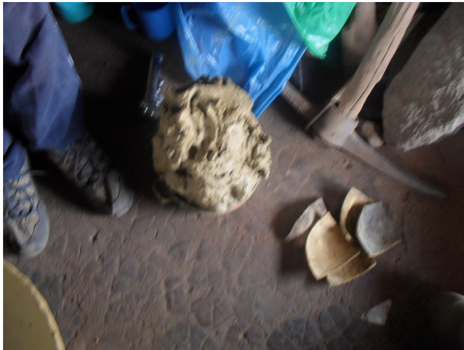
Figure 31: Photos showing wedged clay ready for construction with calabash tool at Fumbisi.
