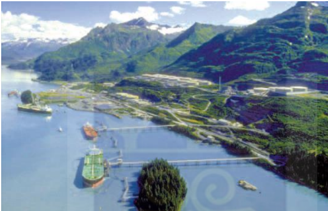
Figure 2.7 On-land treatment station for BW
