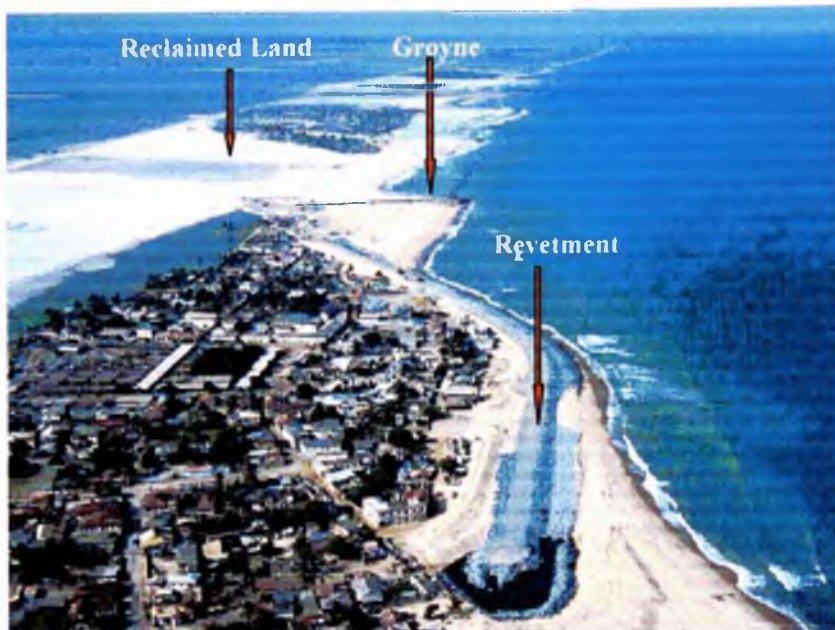
Figure 3. 8 Aerial View of the Keta Sea Defence (GLDD, 2001)
