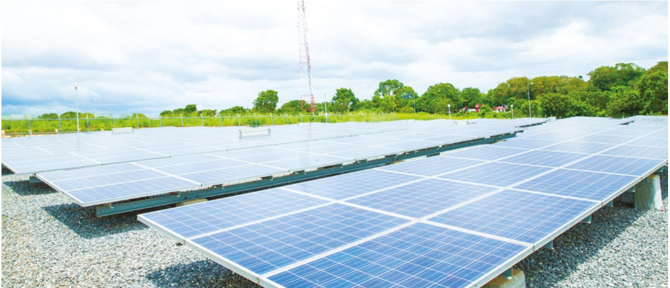
Solar Energy Plant at MNIMR
