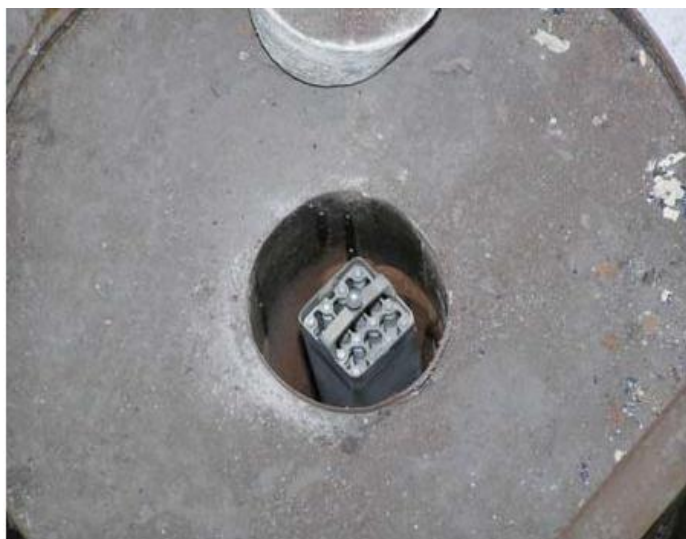
Figure 2.4: View inside one EK-10 drum after plug removal
