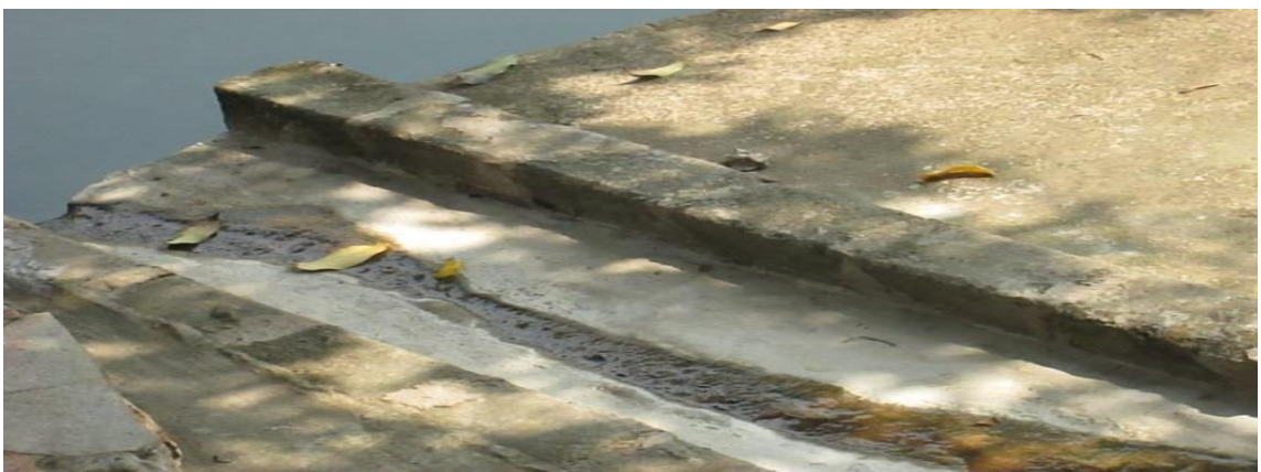
I: Open drain discharging liquid waste from the hotel into the River Volta at Senchi
