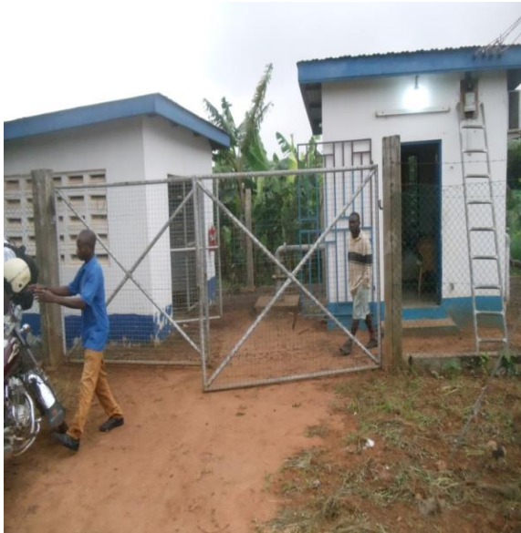
Picture 1: PAWSDB Pump Station (Boi)
