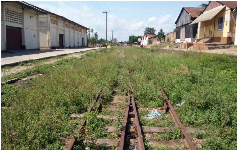
Field Survey 2018: A section of rail track at Nsawam over grown with weeds
