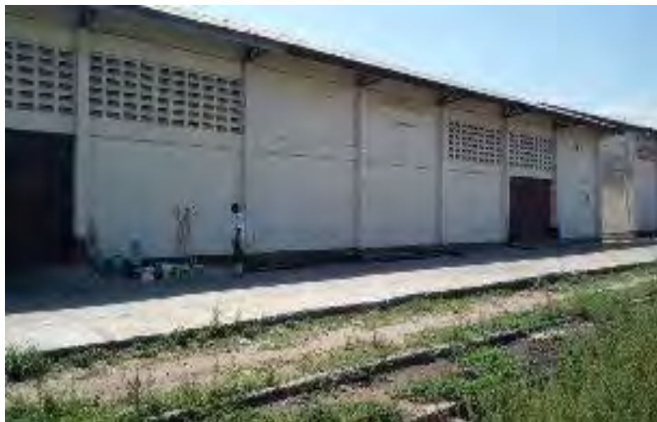
Field Survey 2018. Cocoa House alongside Nsawam railway station overgrown with weeds
